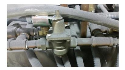
The union is seen at the right of the valve and has right hand threads with an o-ring seal
